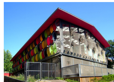
Picture 23 Fawood Children's Centre, Stonebridge.
